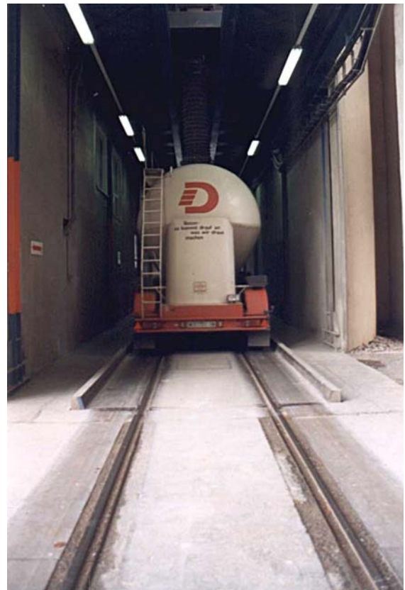
Our combined railway-truck weighbridge "KGW" in action
