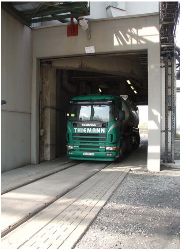
Our combined railway-truck weighbridge "KGW" in action
