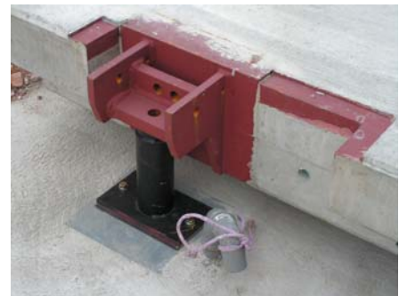
Affixing of load cell dummies for absorption of weighbridge modules
