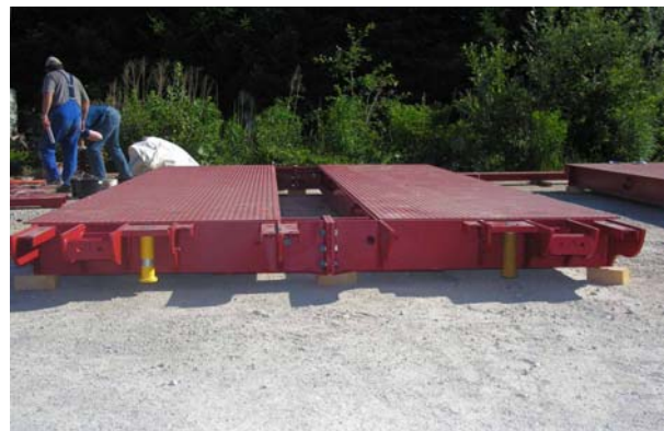
Step 2: Supplied bridge module elements are screwed to form bridge modules
