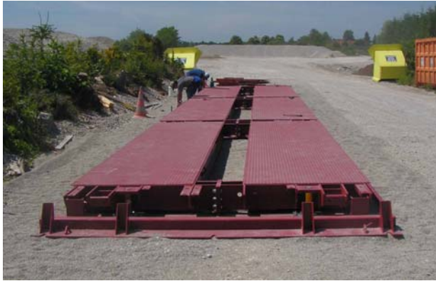
Step 4: Mounting of digital load cells in the weighbridge
