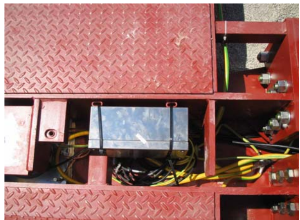
Step 7: Cable running and connection of the digital load cells in terminal boxes. Sealing of the terminal boxes with security stamp.
