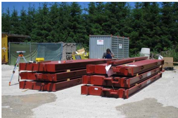
Step 2: Supplied bridge module elements are screwed to form bridge modules
