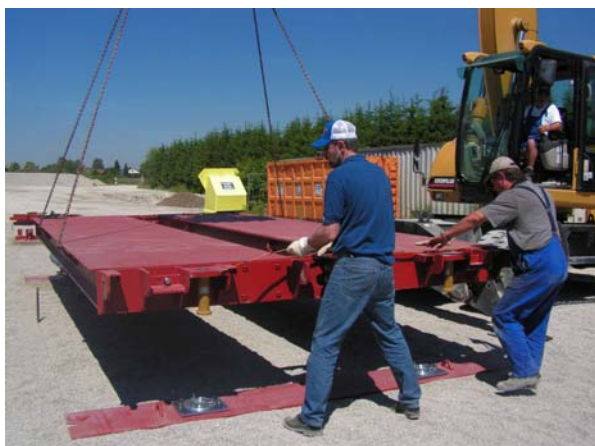
Step 3: Positioning of the bridge modules on steel foundation strips
