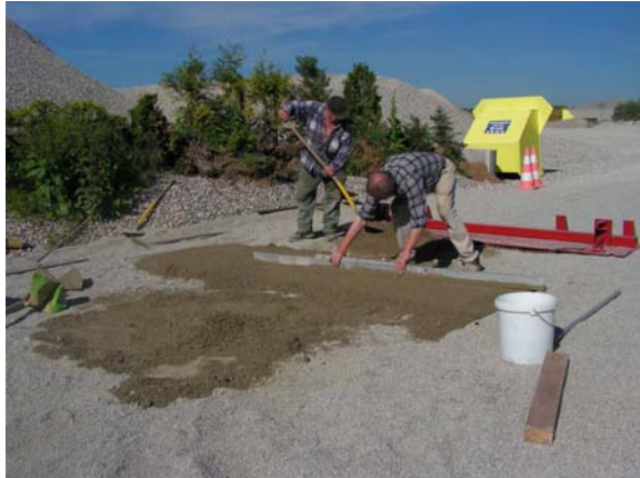
Step 1: On-site preparation of the foundation – important for problem-free erection !
