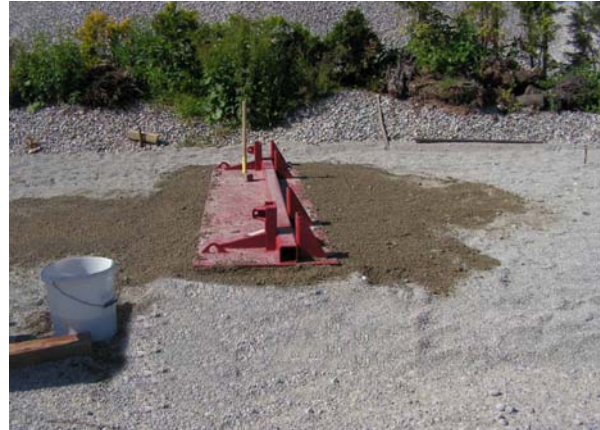
Step 1: On-site preparation of the foundation – important for problem-free erection !
