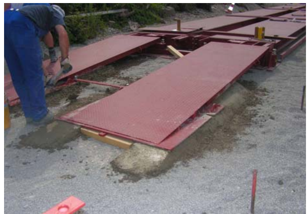
Step 5: Lifting-in and aligning of the run-on ramps. On-site foundation securing for ramps.
