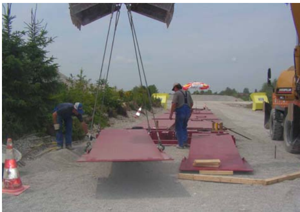
Step 5: Lifting-in and aligning of the run-on ramps. On-site foundation securing for ramps.
