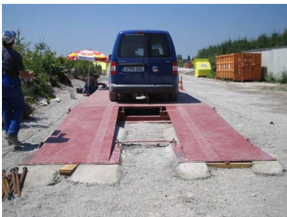
Step 8: Adjustment of the weighing indicator and test with reference weight (e.g. vehicle, weighing document print-out trial)
