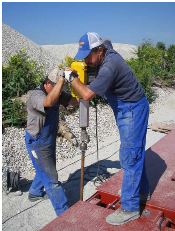
Step 5: Lifting-in and aligning of the run-on ramps. On-site foundation securing for ramps.
