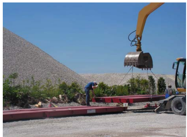
Step 3: Positioning of the bridge modules on steel foundation strips
